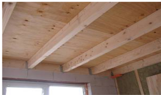
(a) Joist floor [19]
