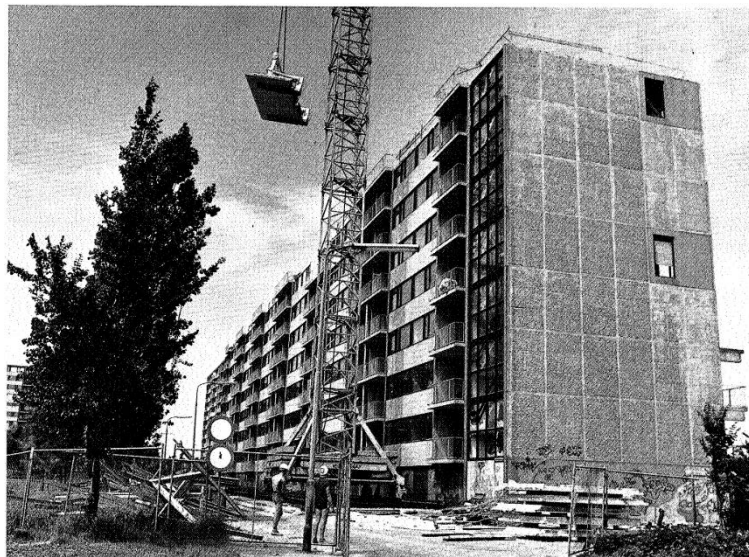
Figure 6. Deconstruction of an apartment building in Middelburg [25].
