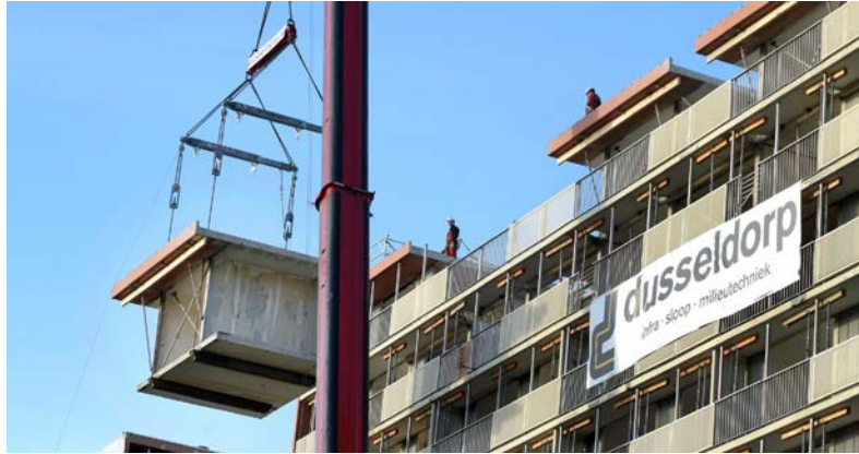
Figure 7. Lifting out of prefab apartment cells [29].
