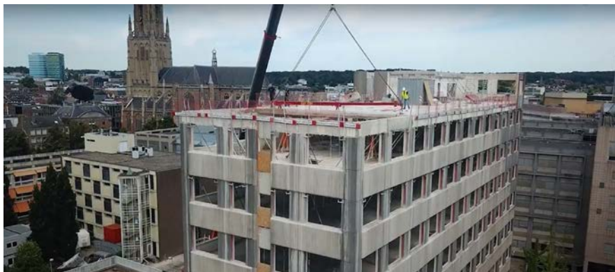
Figure 8. The Prinsenhof A building during deconstruction [32].
