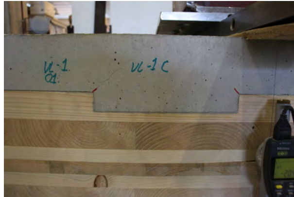
(a) Hairline crack at N2
