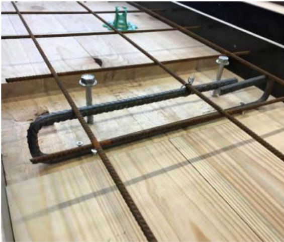
(b) Specimen before pouring of the concrete
