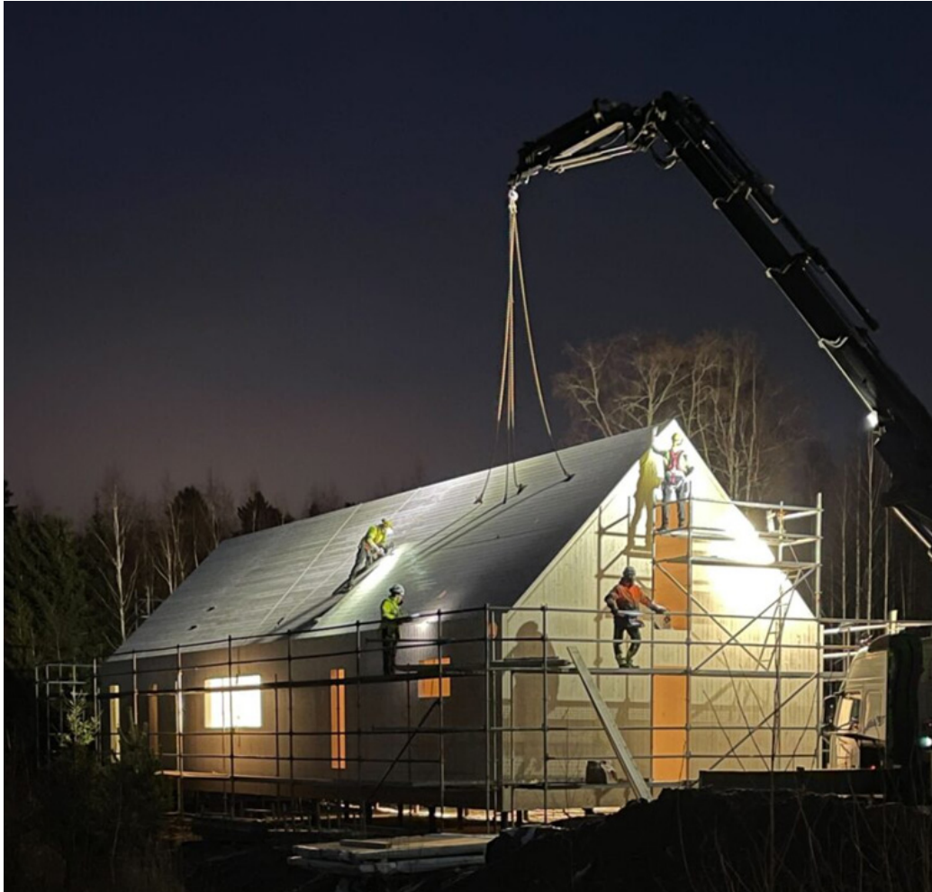
Figure 9: CLT dwelling by Asumma in construction (Mela, 2013)
